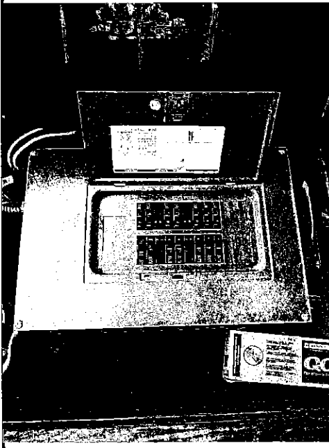
Upper level, second floor 125 amp electrical panel replaced.
