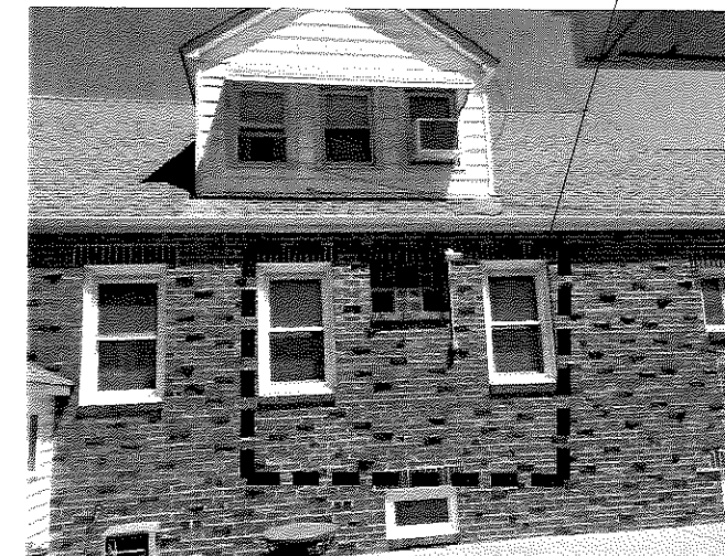
EXISTING REAR FACADE - TO RECEIVE NEW SLIDING DOOR
